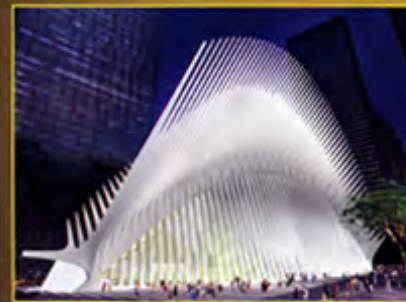
The World Trade Center Port Authority Trans-Hudson Transportation Hub was designed by world-famous and celebrated Spanish architect Santiago Calatrava.
